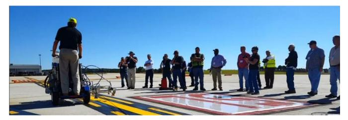
The paint removal demonstration(s) has generally been performed on the marking that will be replaced the following afternoon by the AirMark thermoplastic (provided free of charge); several host airports choose a busy taxiway intersection for AirMark installation to evaluate the durable material's life. A NOTAM citing non-standard markings may be required overnight prior to the AirMark sign installation the following afternoon.
